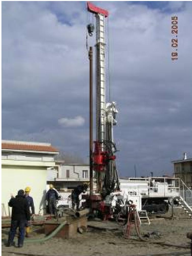
**Fig. 3.4-1 Drilling mast**
